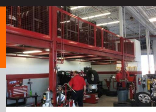
BeastWire RailGuard is a full handrail system including a wire mesh infill and optional kickplate, using all standard BeastWire components.
