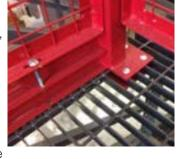
growth plates can be cut and notched in the field, as required.
